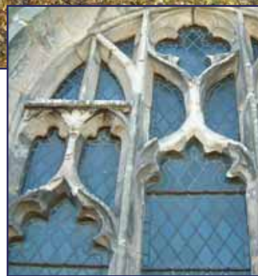
The stonework is crumbling, the metalwork has corroded and the glass is loose.
