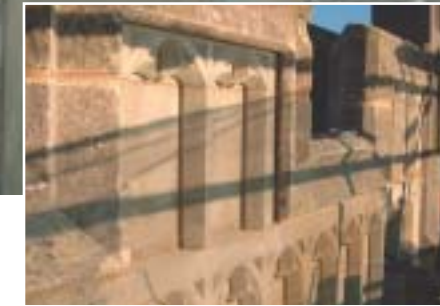
Top: A section of new stone work waits to be finished.
