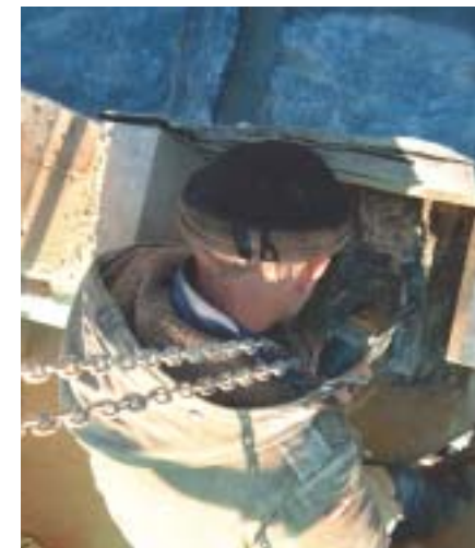
Outside the new timber work is attached to the stone work.
