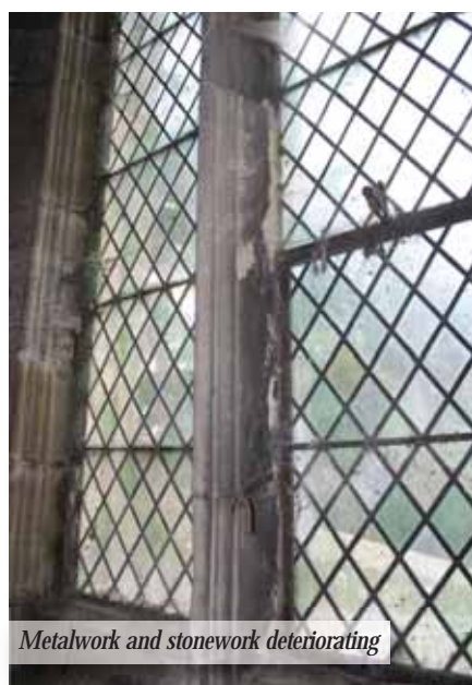
The masonry is crumbling away and the metalwork that holds the glass in place is corroding.
